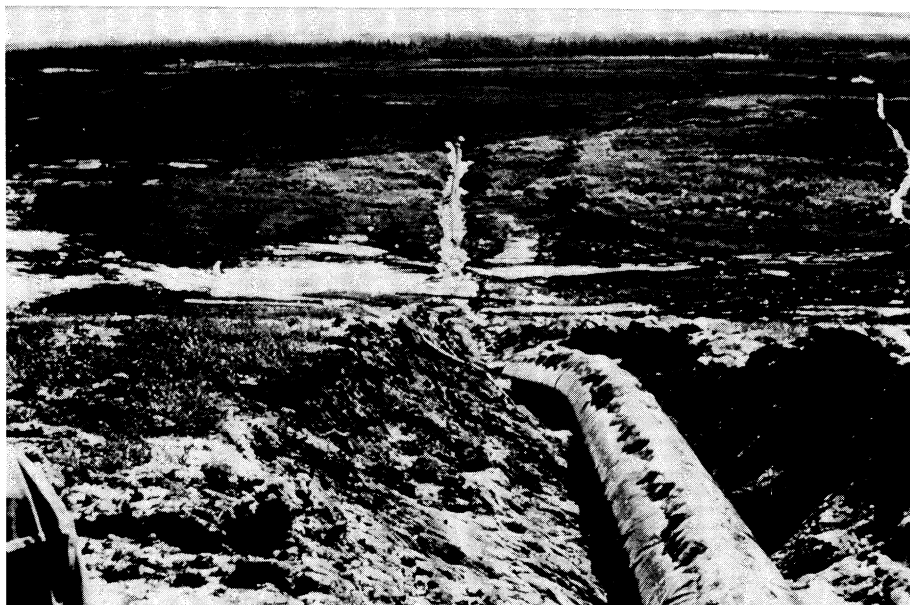
Figure 2. Large pipeline exposed by erosion following freezing, heaving and thawing of near surface layers above permafrost (Siberia). Photograph by E. D. Ershov.
